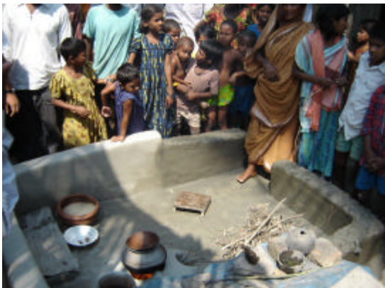
New barrier around cooking area in a Raiganj Area home.
